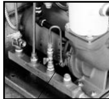
Pump seal cooling line Figure 5.2D
