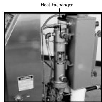
Heat Exchanger Figure 6.1G
